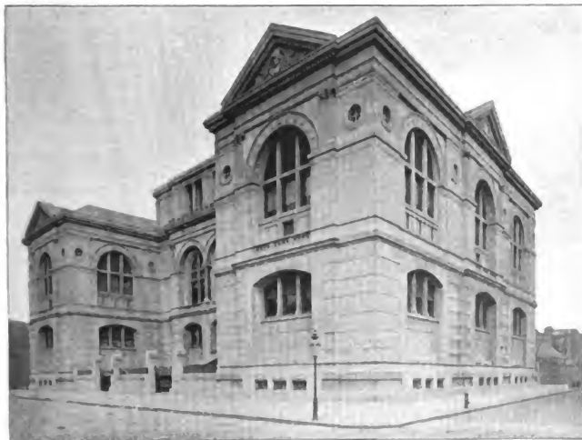
LENOX LIBRARY, FIFTH AVENUE, 70TH AND 71ST STREETS.
